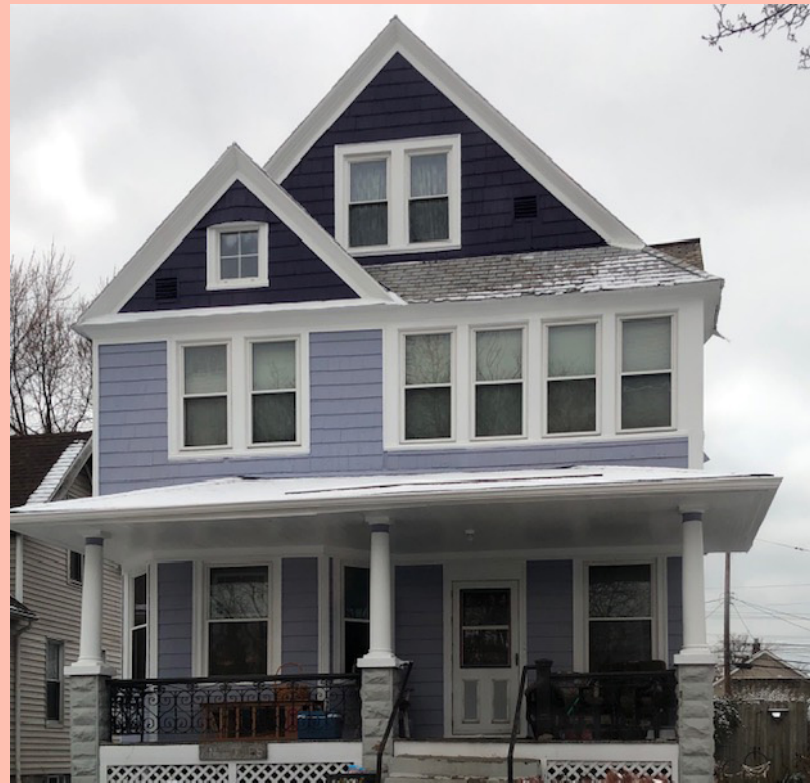
Citizens Paint Program provided supplies for this exterior
