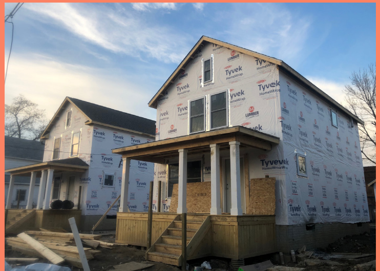
CHN Lease Purchase construction on West 85th Street
